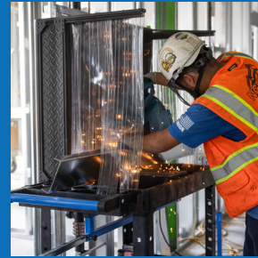
3-sides of protection from sparks and debris
